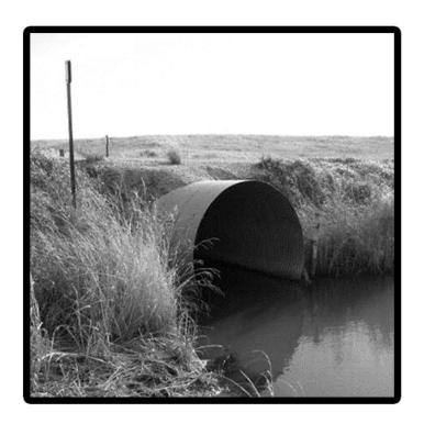
A culvert should be installed in such a way that the bottom of the structure is at least 6 inches below the streambed to allow for fish passage and to mimic the natural stream bed.
