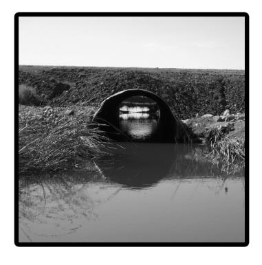
Implement comprehensive and effective sediment and erosion control measures to the greatest extent possible during installation so that rip rap and other fill material do not impede the flow of water from the entrance and exit of the culvert.
